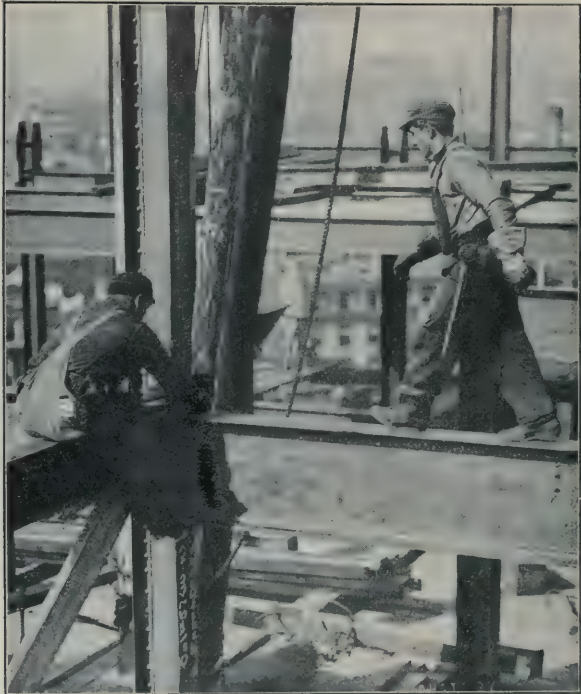
JOINING THE "ANGLE BEAMS" ON A "SKYSCRAPER"
